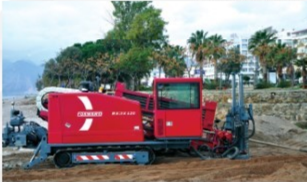
Laying of water inlet pipe for Antalya Aquarium in Turkey
