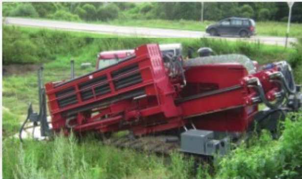
Construction of water supply and sewerage systems
