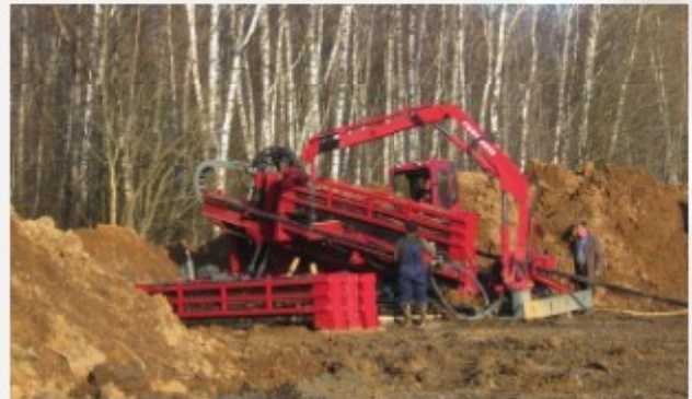
Construction of water supply system
