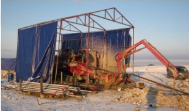
Crossing under Kama river
