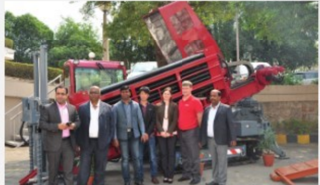
Laying of pipeline in New Delhi, India
