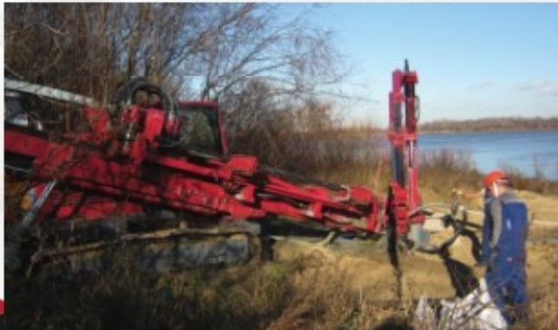
Crossing under Oka river
