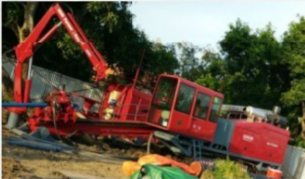
First drilling in Indonesia
