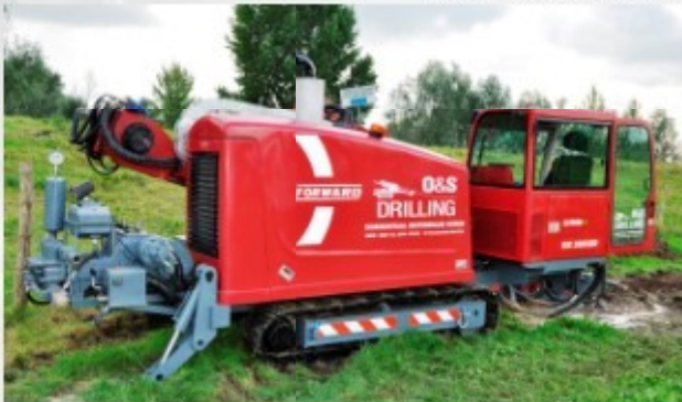
Laying of fiber-optic cable in Netherlands
