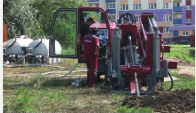
Universiade facility in Kazan
