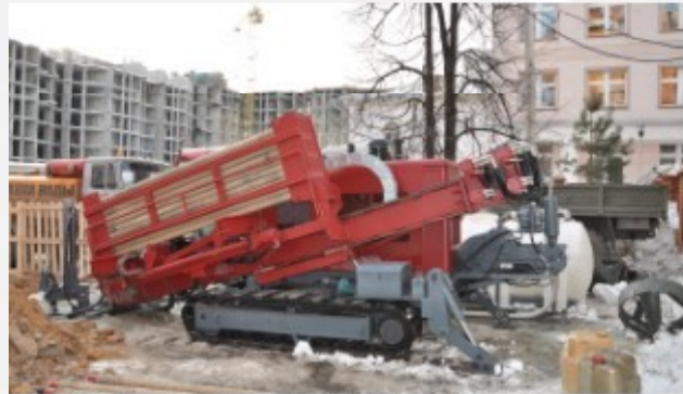
Construction of water pipeline in St. Petersburg
