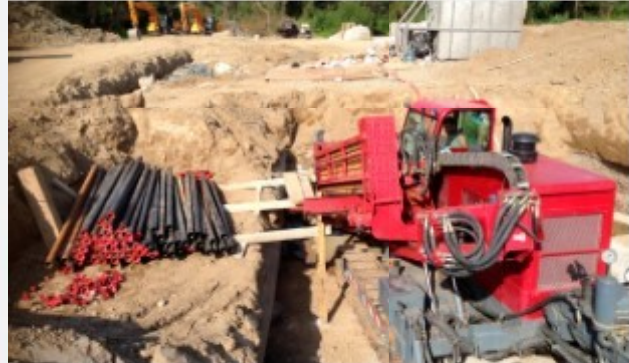
Construction of gas pipeline near Istanbul, Turkey
