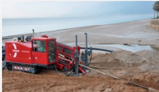
Drilling in Antalya, Turkey
